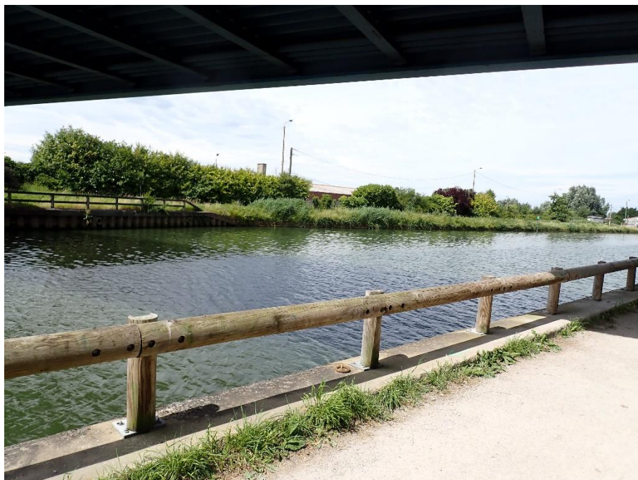
Figure 7 : Upstream site of the Aa at Saint-Momelin
