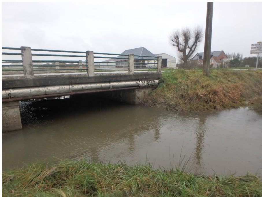
Figure 33 : Upstream site on the Canal de Retz River at Monchaux (Quend)
