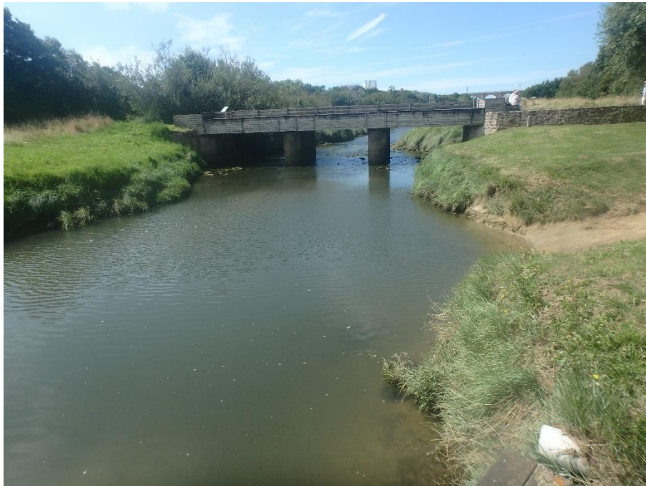
Figure 18 : Downstream site on the Wimereux River at Wimille
